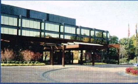
Headquarters in St. Louis, Mo.
